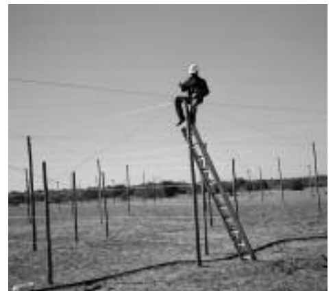
Community member Ruben Makgabo hammers tire treads to protect net house poles at Diretsogetse.
