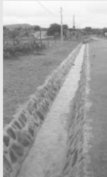
Storm water drainage system built by Matlala, Ragalakane, Matlamyane and Tabane.
